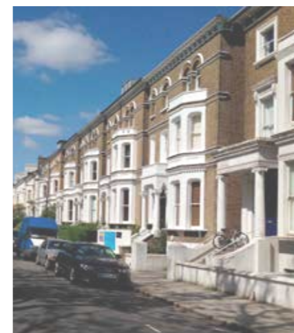
Terrace to north of Lancaster Grove
