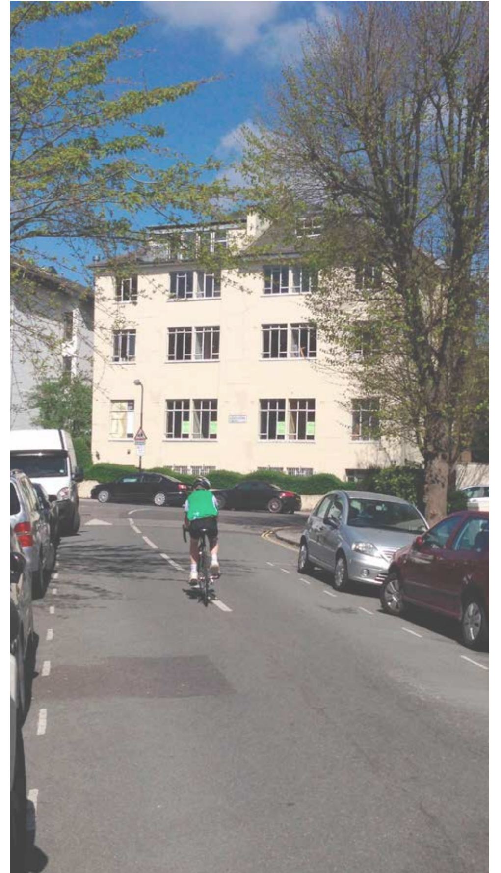
Clifford Pugh House, Lancaster Grove, NW3
