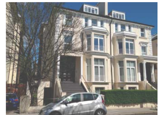
Adjacent terrace 9-15 Lancaster Grove
