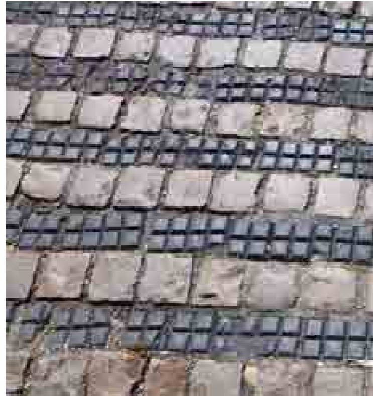
Mixing blue stable blocks with granite setts
