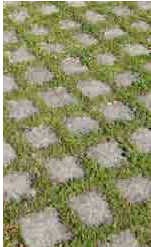
Setts layed with spaces to allow water percolation
