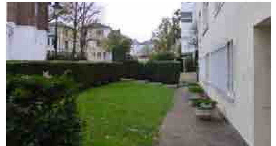
View of the front garden of the existing property
