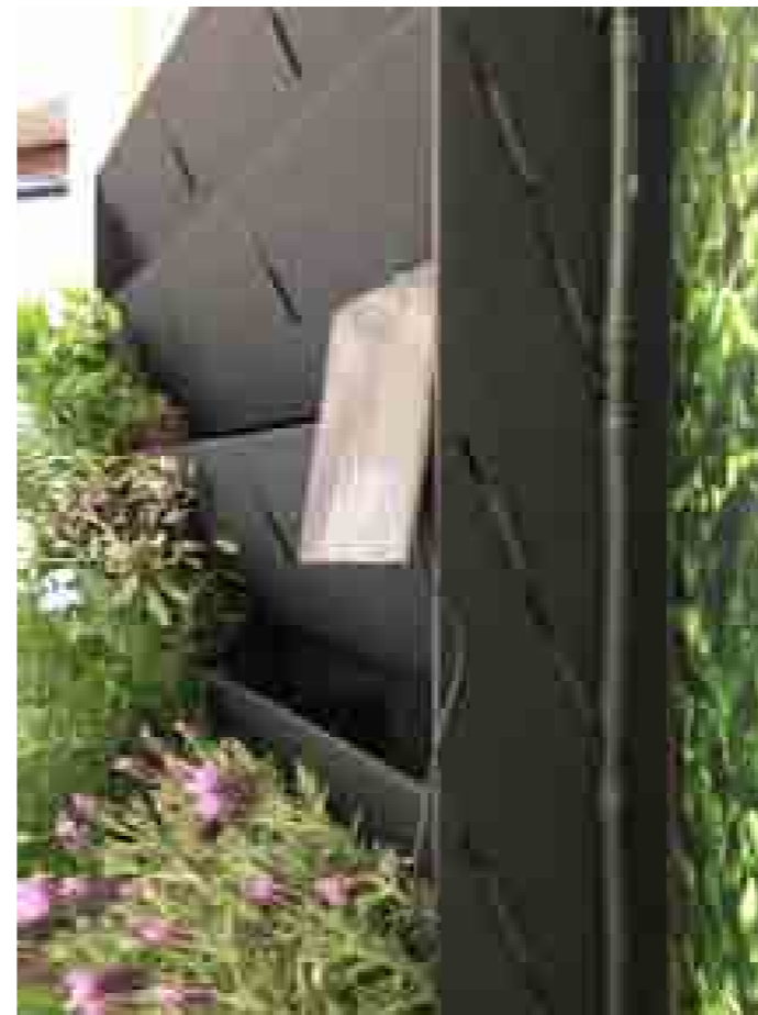
Treebox greenwall system used as vertical rain garden at rear to intercept roof water
