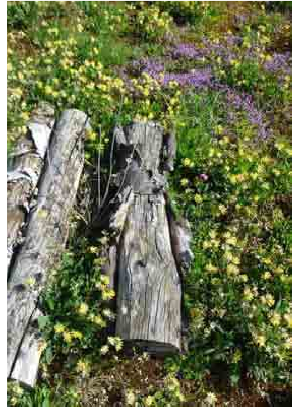
Log pile of a living roof
