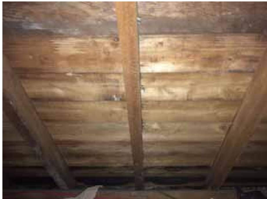
Interior of attic space.
