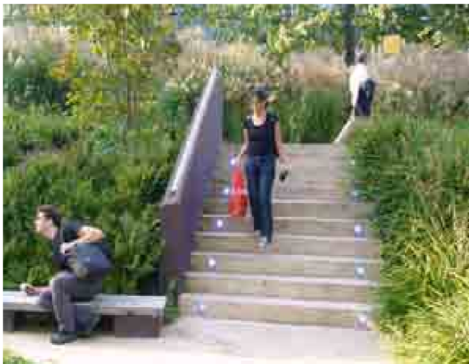
Low key LED lighting for stairs, floor washing with bollard lighting in planting and LED spots for some strategic plants
