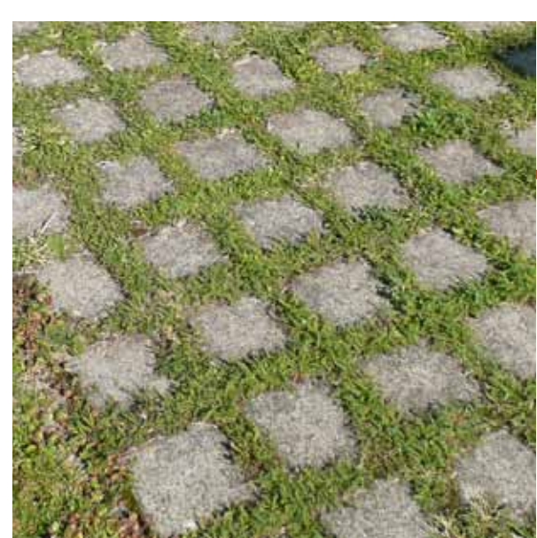
Reclaimed light grey granite setts
