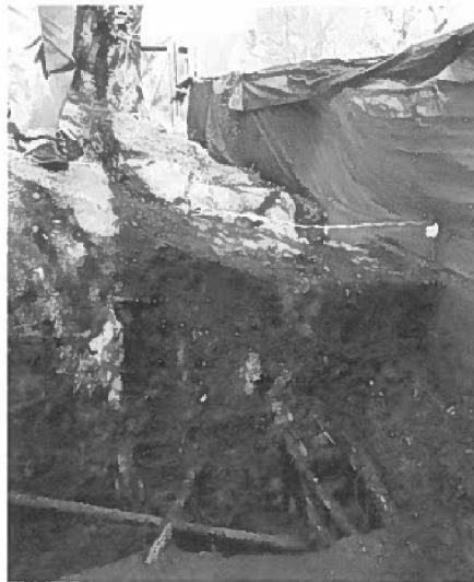
Photo 4. Large bundle of large roots immediately behind the existing retaining structure
