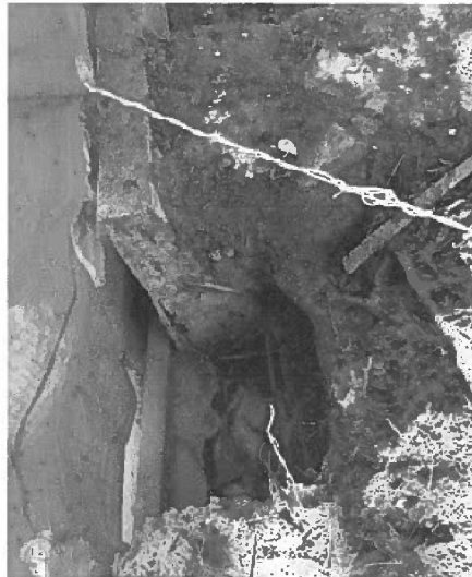
Photo 6. Very large root just behind the retaining structure.
