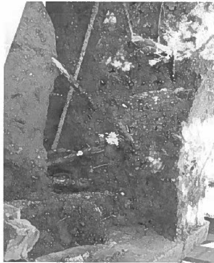
Photo 6. Very large root just behind the retaining structure.
