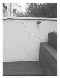
There is sign of extensive movement of the party wall and visual signs of cracking. This is both historic and recent. The wall has had cracks repaired in the past on more than one occasion as can be seen by the new plaster and painted areas. Many of these cracks are right through the brickwork and evident on the opposite side.
