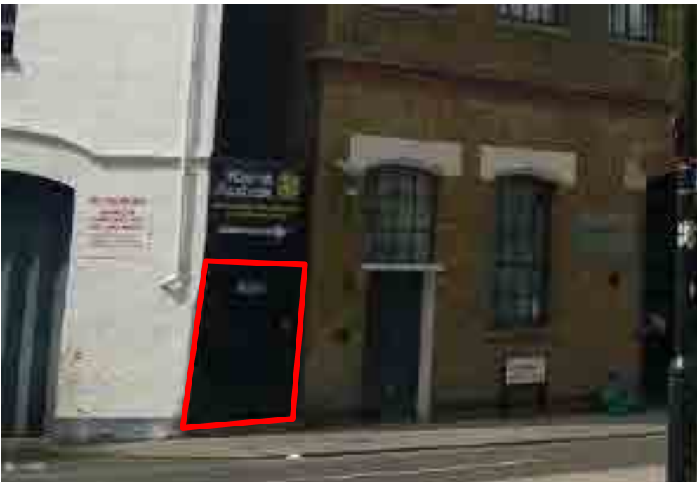
Photograph 2.5: Locked passageway to small rear yard (between buildings)
