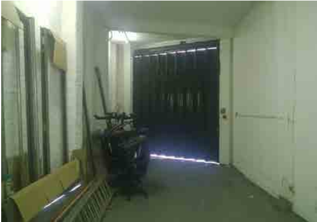
Photograph 2.7: Loading bay (no evidence of staining)
