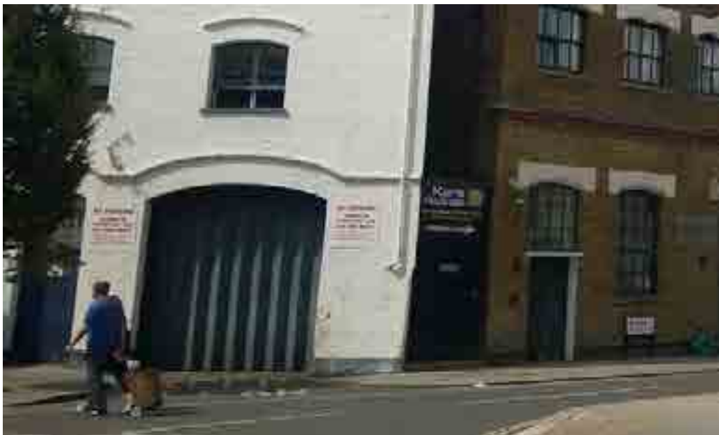
Photograph 2.3: Shutter door/unloading bay associated with 256 Belsize Road
