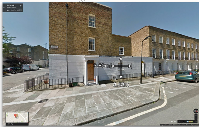
11 Penryn Street Three-storey rear extension (basement, ground and first) behind garden wall.
