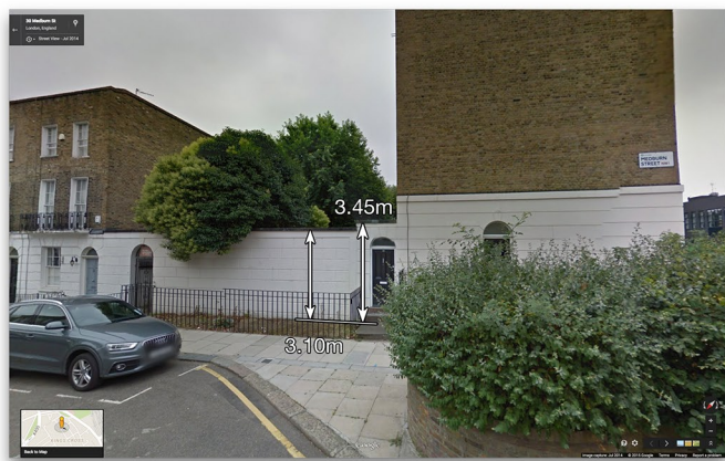
30 Medburn Street Two-storey rear extension (basement and ground) behind garden wall.
