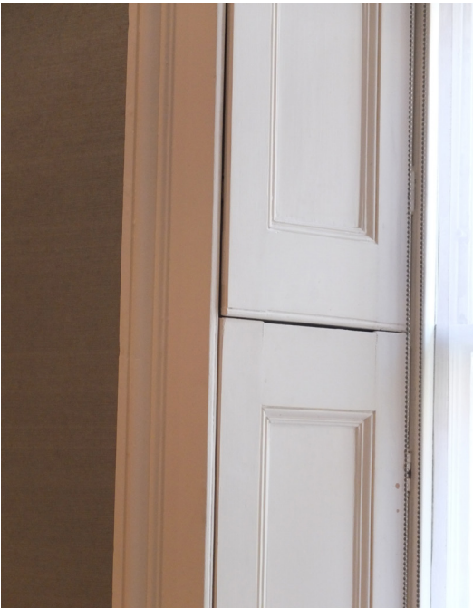
Above: Panelled shutters to sash windows.
