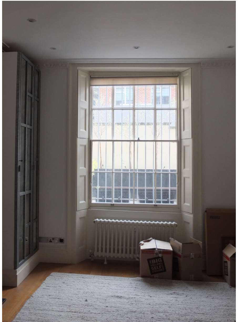
Top Right: Six over six pattern sash windows to front room at Ground Floor (overlooking street).
