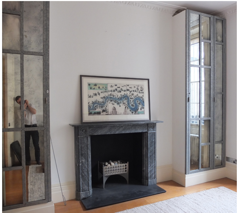
Bottom Right: Mirrored joinery units to either side of chimney breast in rear room. Grey marble fireplace.
