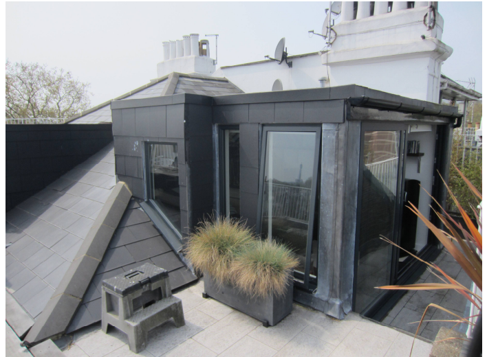
ROOF VIEW FROM TERRACE
