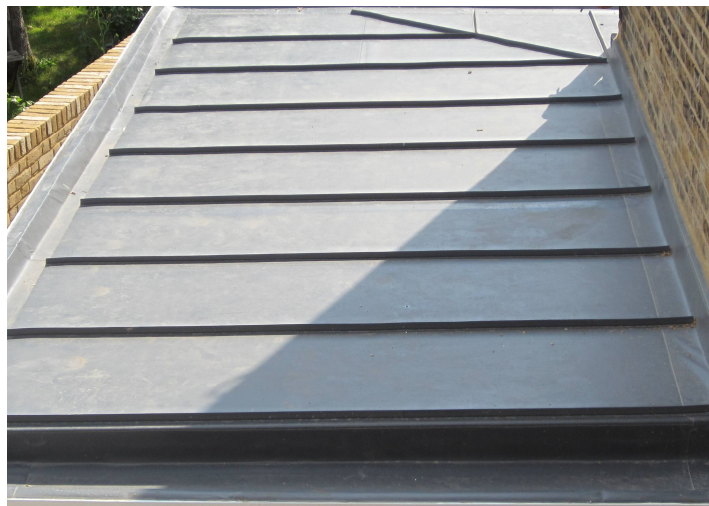
SINGLE PLY MEMBRANE ROOF - TYPICAL
