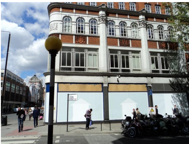
Figure 3 - Store Street Facade
