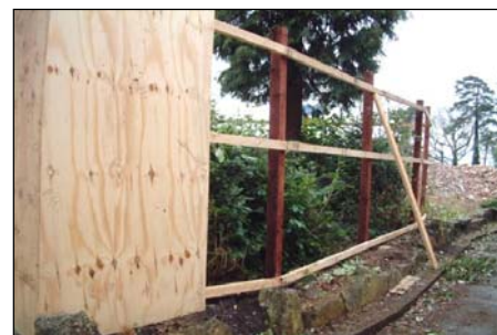
Photo 4: Board specification on secure wooden posts is a suitable alternative to the standard braced scaffold design.
