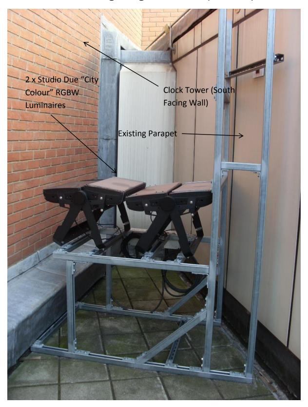
Studio Due City Colour Luminaires mounted on Uni Strut framework at the base of the Clock Tower on Level 3 behind existing parapet.
