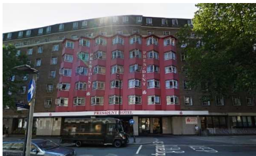
Figure 2 – Guilford Street façade – painted off-shutter concrete proposed for removal
