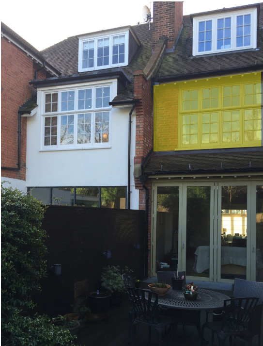
Rear elevation. Wall (highlighted in yellow) to be moved outwards to align with neighbours wall creating a dormer window at intersection with roof
