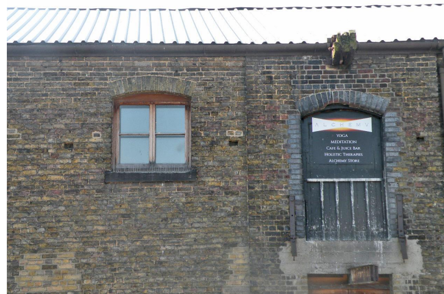
Figure 9 Provender Store north elevation showing modern profiled metal sheet roof covering.
