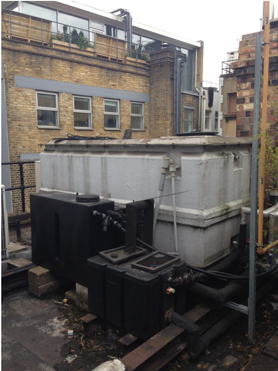
Photograph Two: Tank and equipment to be removed from roof level
