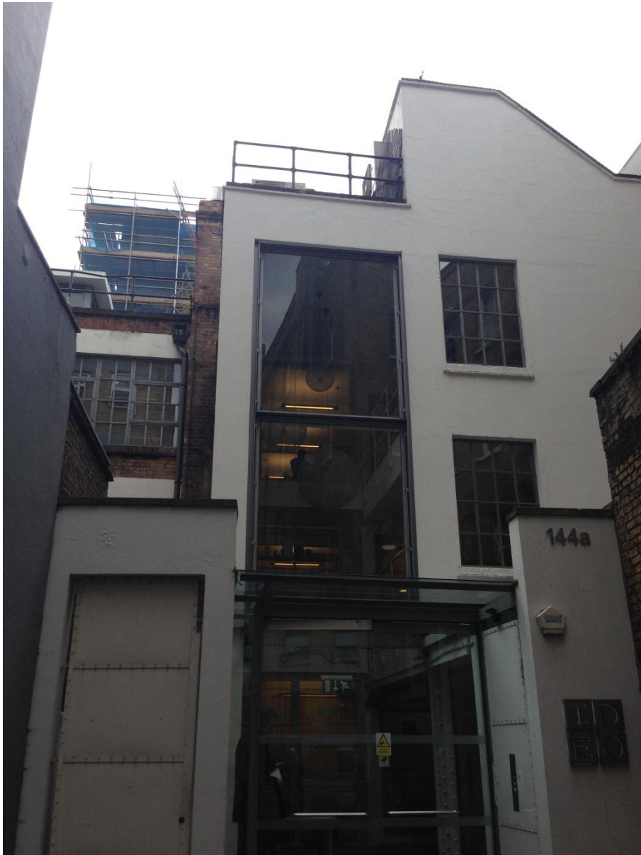
Photograph One: View from Clerkenwell Road entrance.
