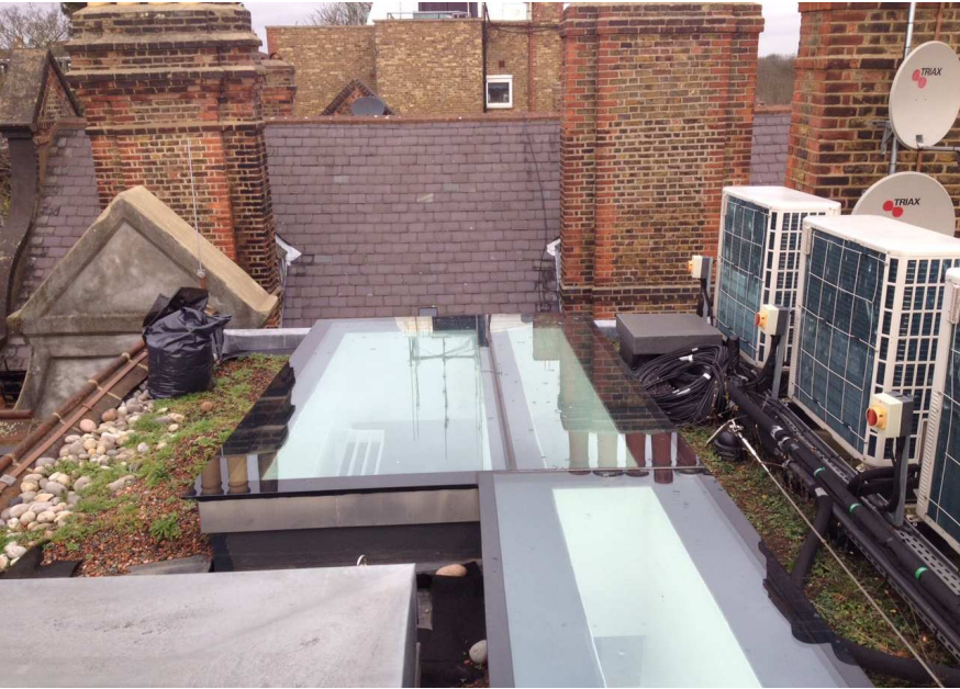
Flat roof lights
