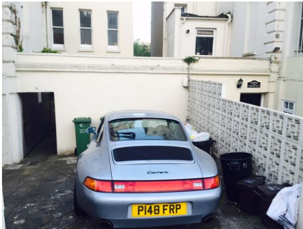
Existing front elevation of garage
