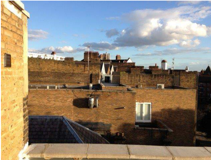
1. North to South View
