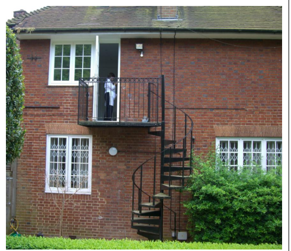
EXISTING BALCONY- IMAGE 01
