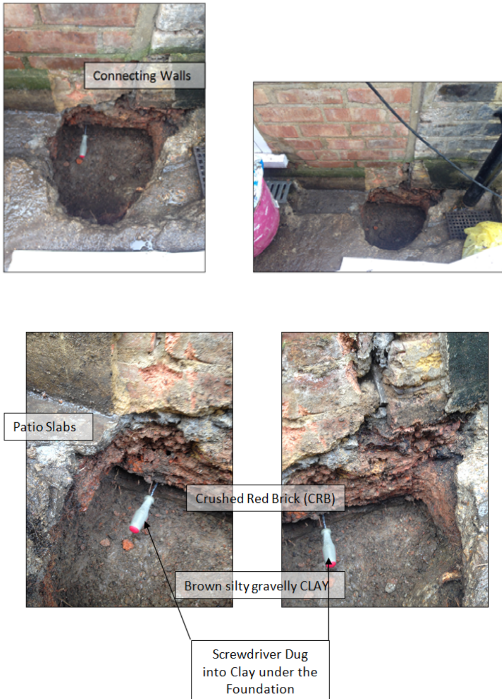
Figure 6 Trial Pit Photographs
