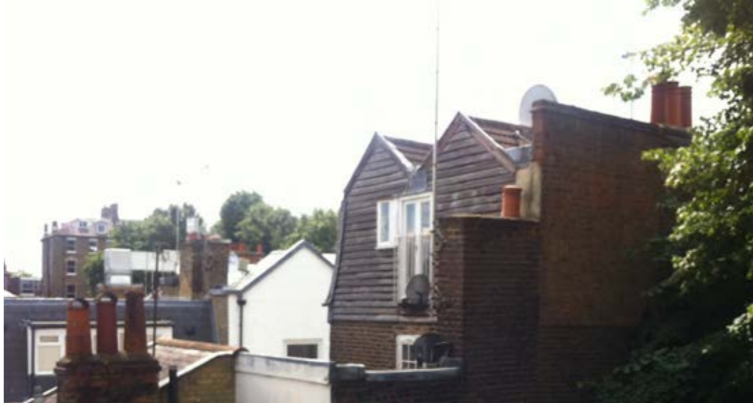
1. View of 6 Perrins Court loft extension with weatherboard gables
