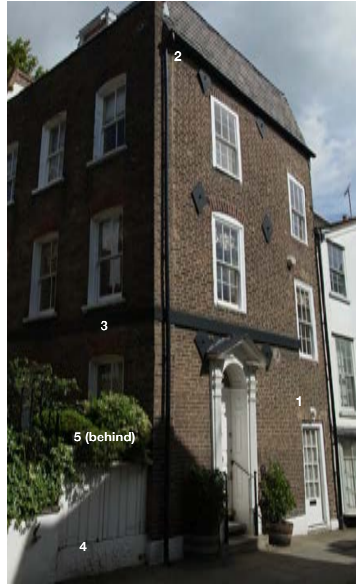
1. Mismatching colours of the upper two brick courses and the pointing indicate the extent to which we believe the original Georgian window opening was infilled
