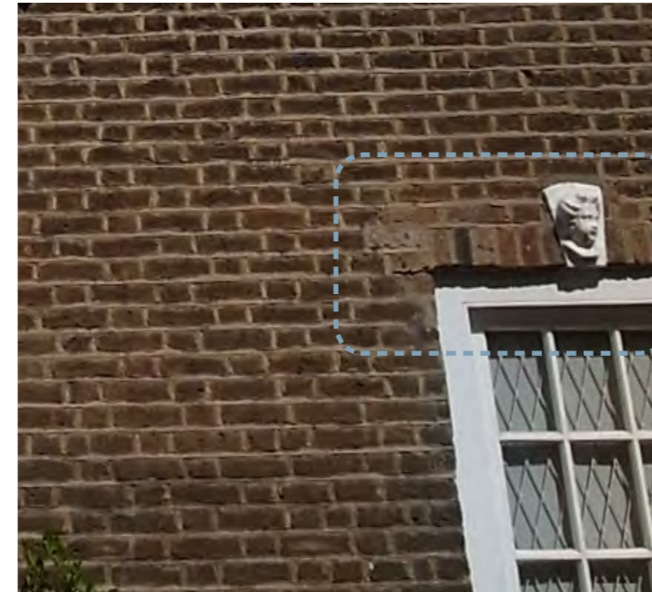
1. Mismatching colours of the upper two brick courses and the pointing indicate the extent to which we believe the original Georgian window opening was infilled
