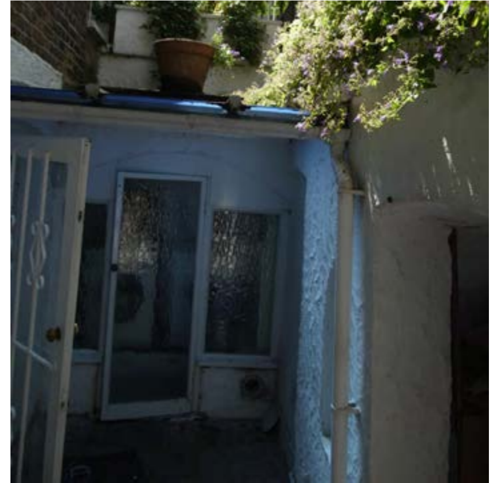
6. Enclosure to underside of existing masonry arch. Existing Glass Canopy.
