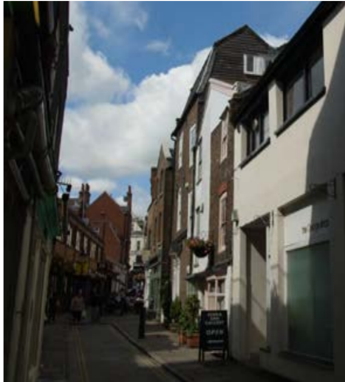
3. View of 6 Perrins Court from Hampstead High Street illustrating the existing weatherboard gable ends.
