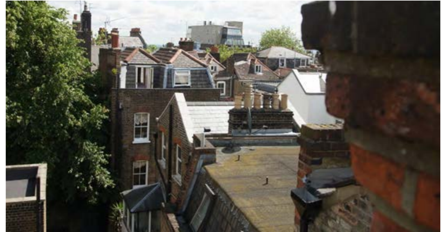
4. View of 6 Perrins Court roof alterations and terrace
