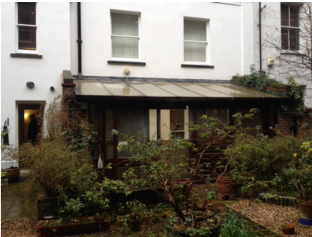
Rear Facade Lower Ground Floor
