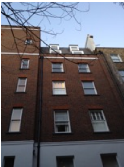
Rear Facade of Ground Floor and above
