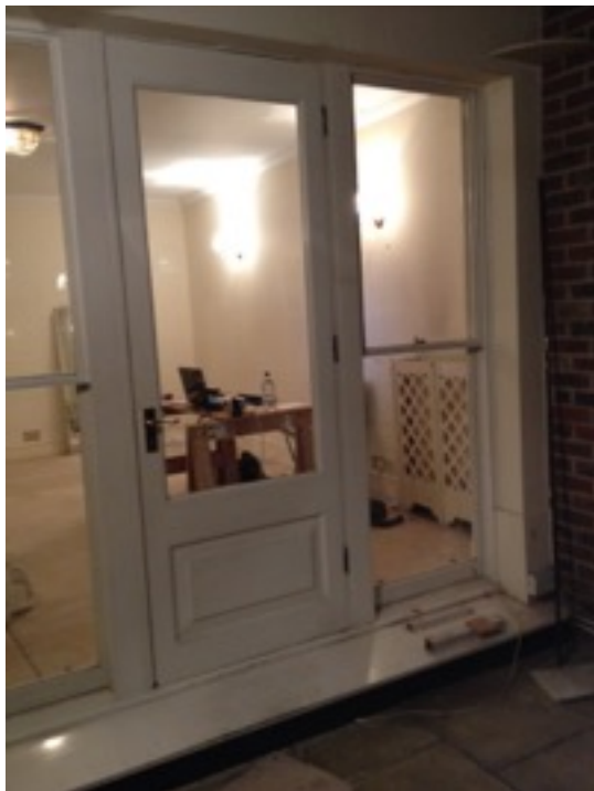
Existing Timber panel door between living and existing conservatory
