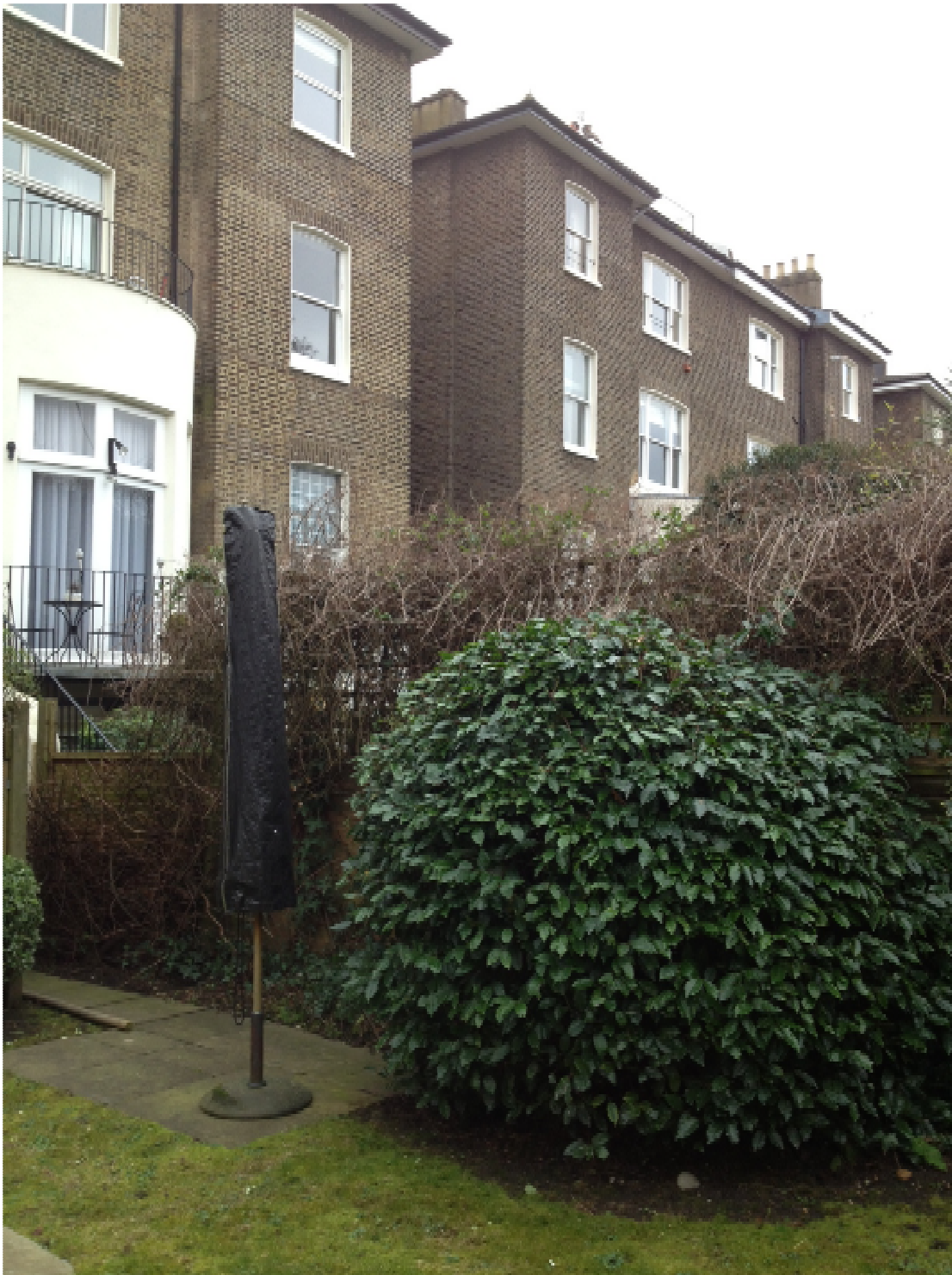
View of shared boundary with No. 25
