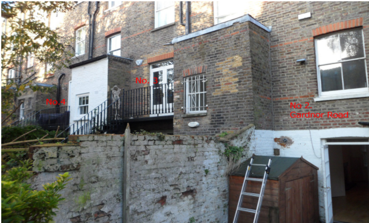
Rear of the properties No. 2, 3 and 4 showing first floor terrace balconies.
