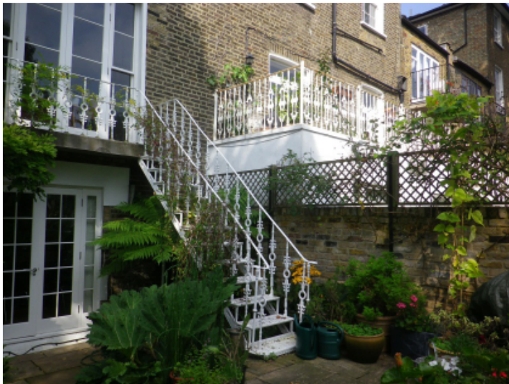
Photo 4: Facing towards No.6 Parkhill Road
