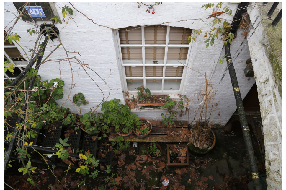
4 Mecklenburgh Street Lower Ground Light Well
