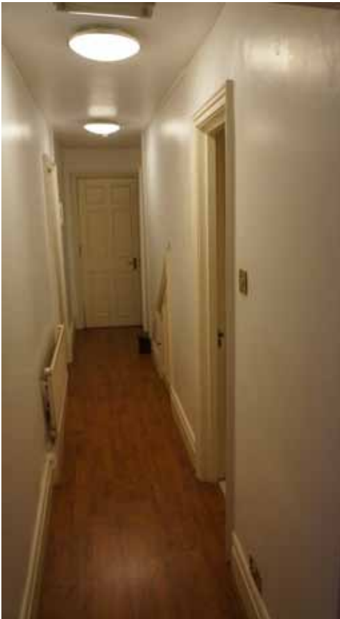
B8. NON-ORIGINAL PARTITIONS
