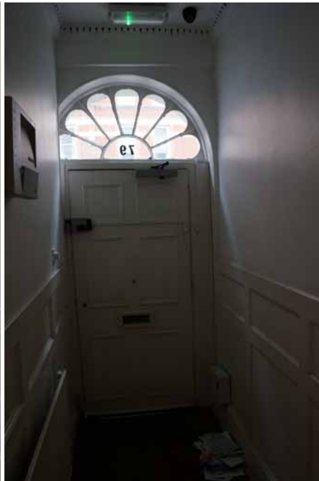
G2.HISTORIC PANELED DOOR WITH ORIGINAL FAN LIGHT ABOVE
