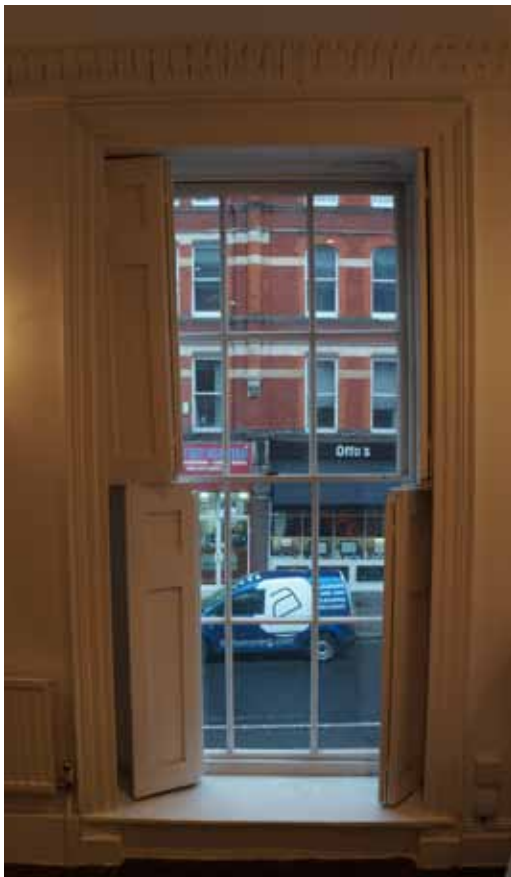
F1. NON-ORIGINAL SASH WINDOWS WITH SECONDARY GLAZING
