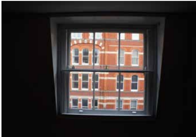
T1. NON-ORIGINAL SASH DORMER WINDOWS
