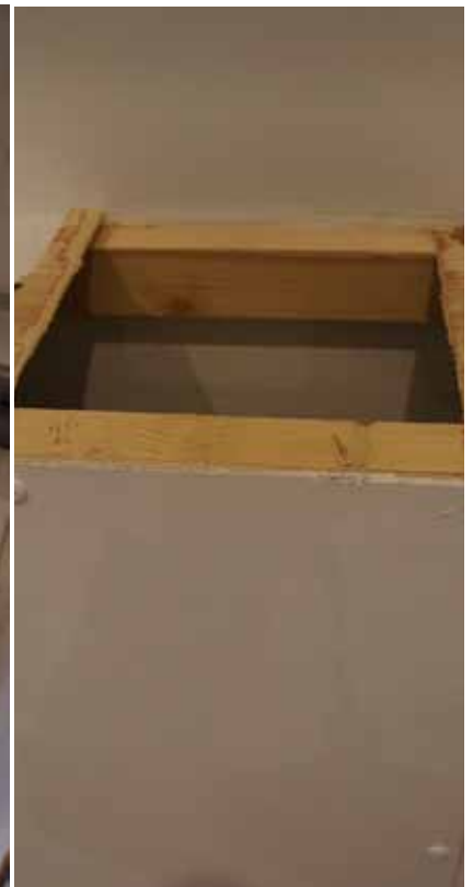
F8. BOXING ENCLOSING SOIL PIPE
