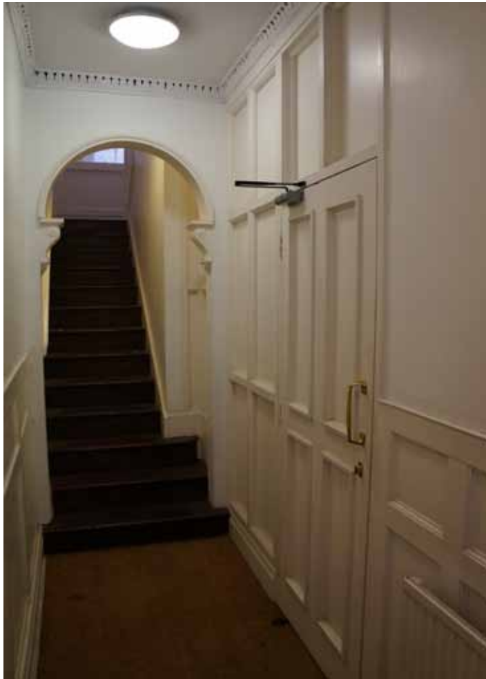
G1.NON-ORIGINAL STAIRCASE AND ARCH
