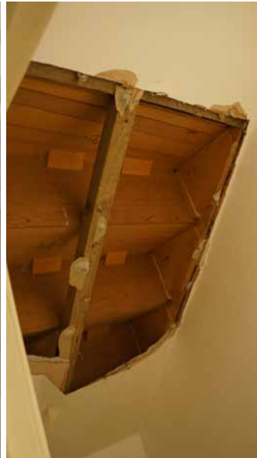
B10. NON-ORIGINAL STAIRCASE
