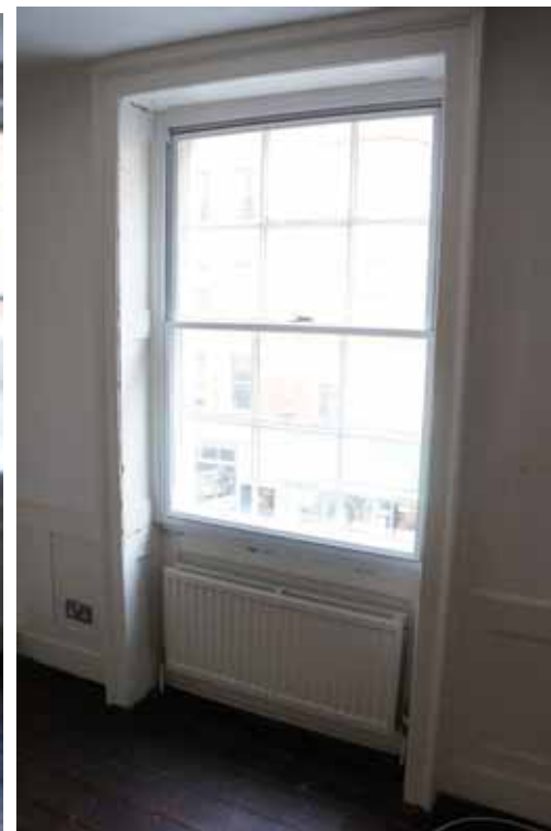
S2. ORIGINAL TIMBER SASH WINDOWS
