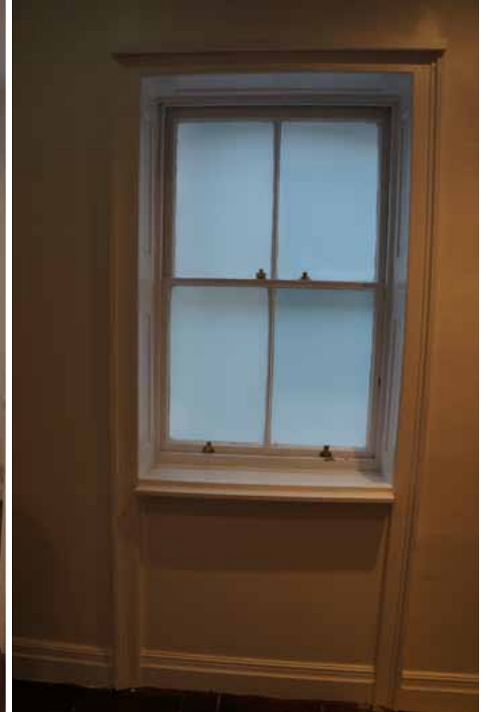
G9.NON-ORIGINAL PAINTED TIMBER SASH FACING COURTYARD
