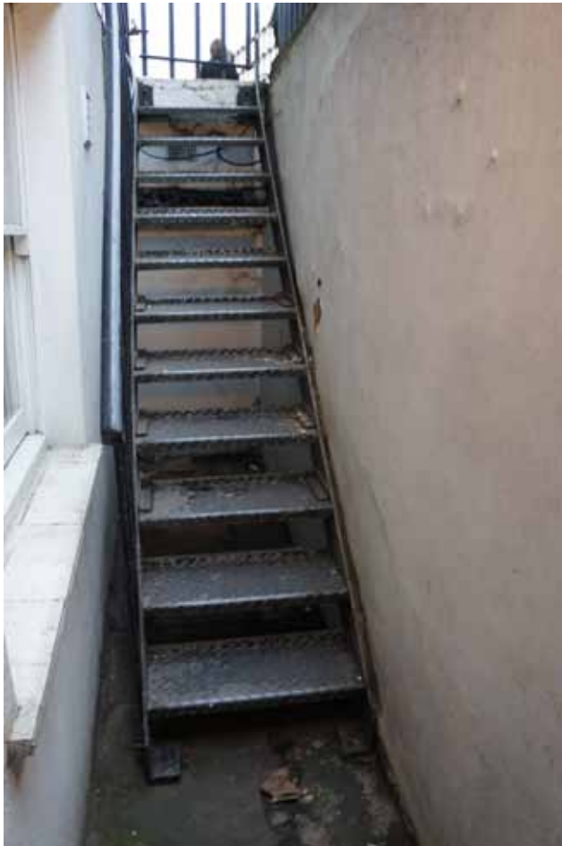
B1. EXTERIOR STEEL STAIRCASE
