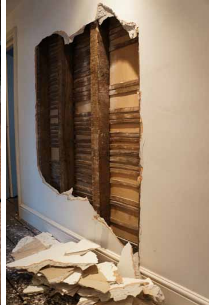
T4. NON-ORIGINAL PARTITION WALL
