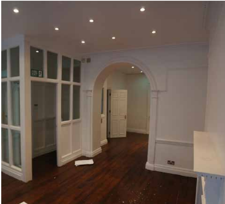
G4.NON-ORIGINAL TIMBER PARTITION AND ARCHWAY
