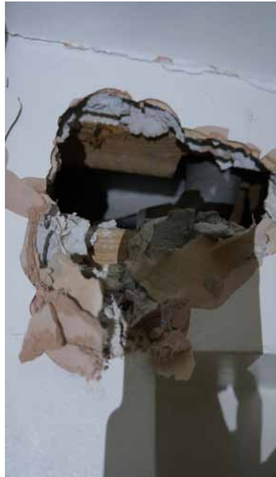
S5. BOXING ENCLOSING DRAINAGE PIPES
