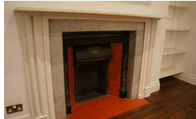
F3. NON-ORIGINAL 19TH CENTURY FIREPLACE AND SURROUND WITH TILED HEARTH
