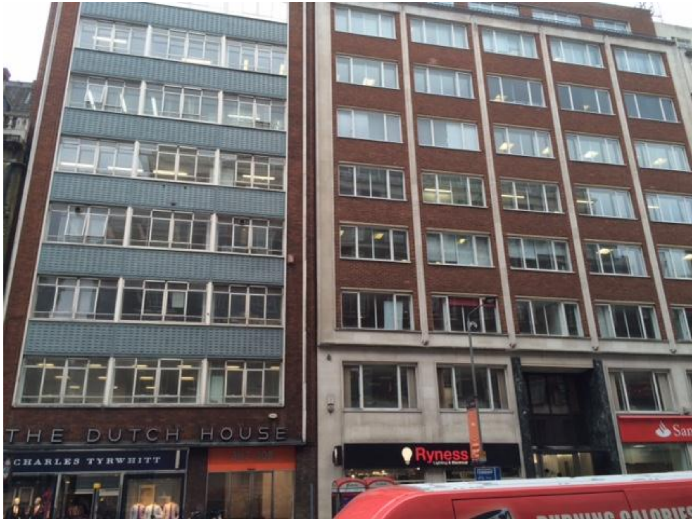
EXISTING FRONT ELEVATION SHOWING BOTH THE DUTCH HOUSE & NORTHUMBERLAND HOUSE – 307-309 HIGH HOLBORN, LONDON WC1V 7LN
