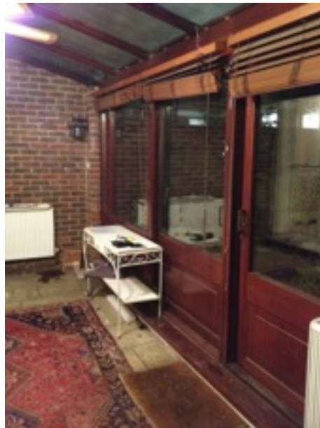
West Side of the existing conservatory and dark timber framed sliding doors
