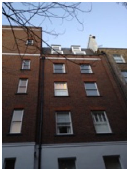
Rear Facade of Ground Floor and above
