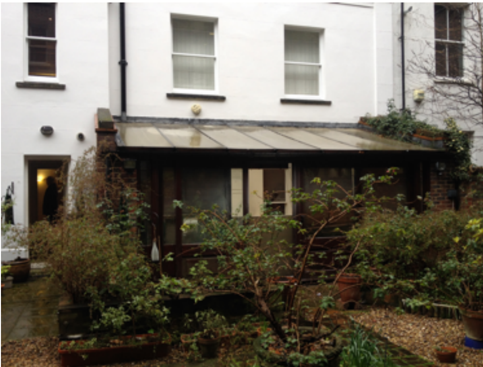
Rear Facade Lower Ground Floor
