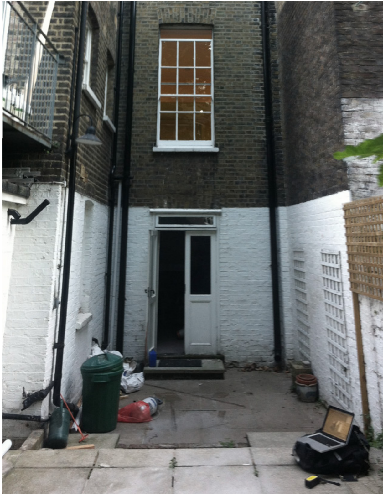
Below: Photograph of rear elevation - 4 Regent's Park Terrace
