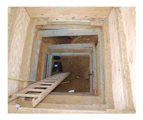
Figure 4 – Typical Underpin Excavation with Supported Sides (Source ASUC Library)
