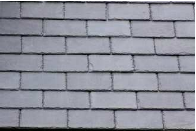
Mansard roof: Traditional slate roof on timber battens
