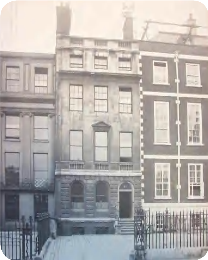
No.65, with No.64 adjacent to the left, in the early 20th century.
