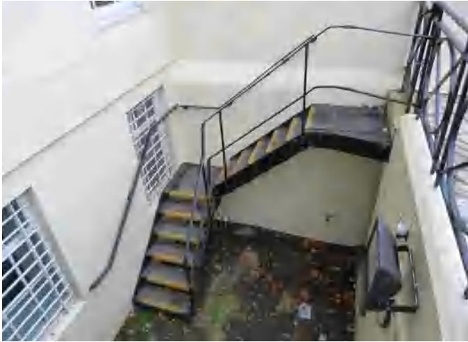
Northern lightwell with modern metal steps
