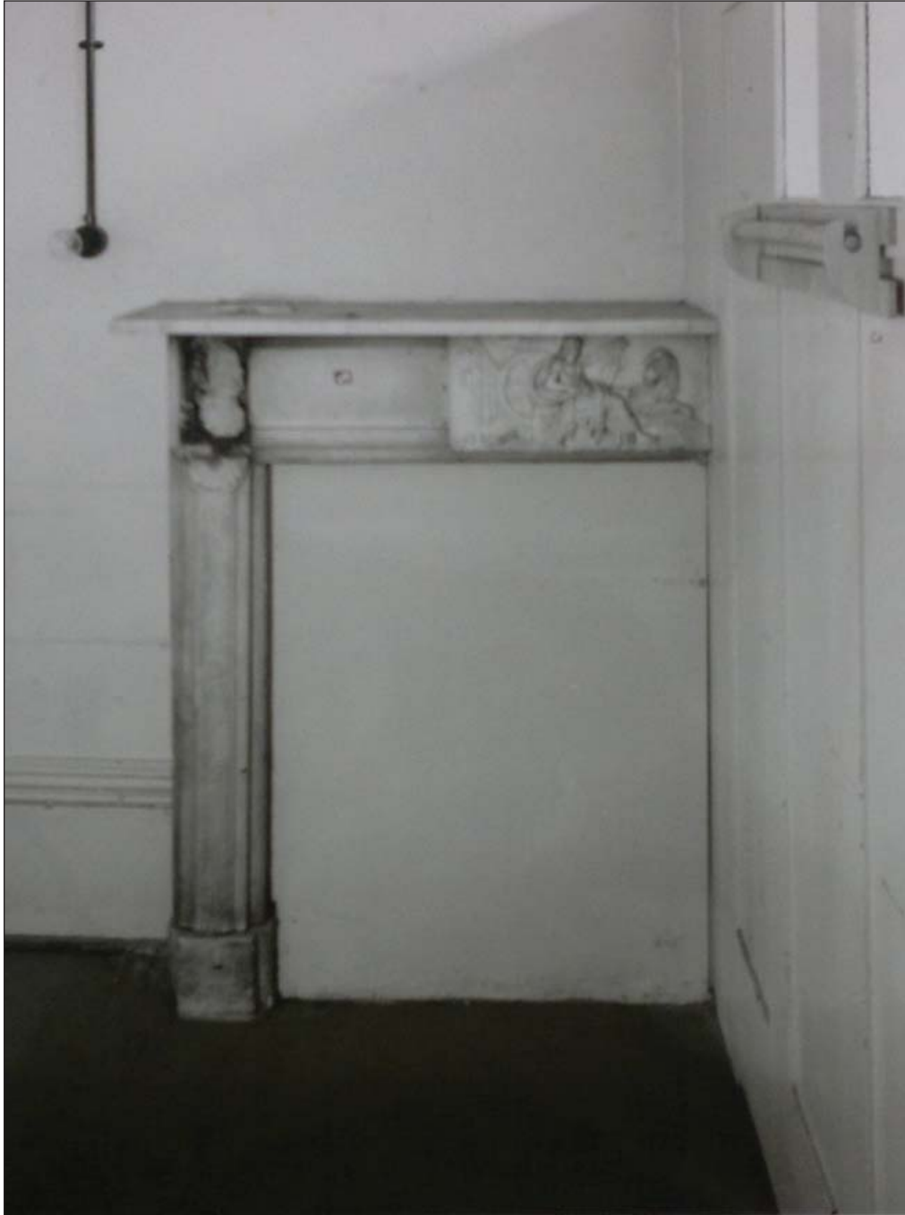
14. First Floor Rear Chimney Piece 1977 (LMA SC/PHL/01/340-53)
