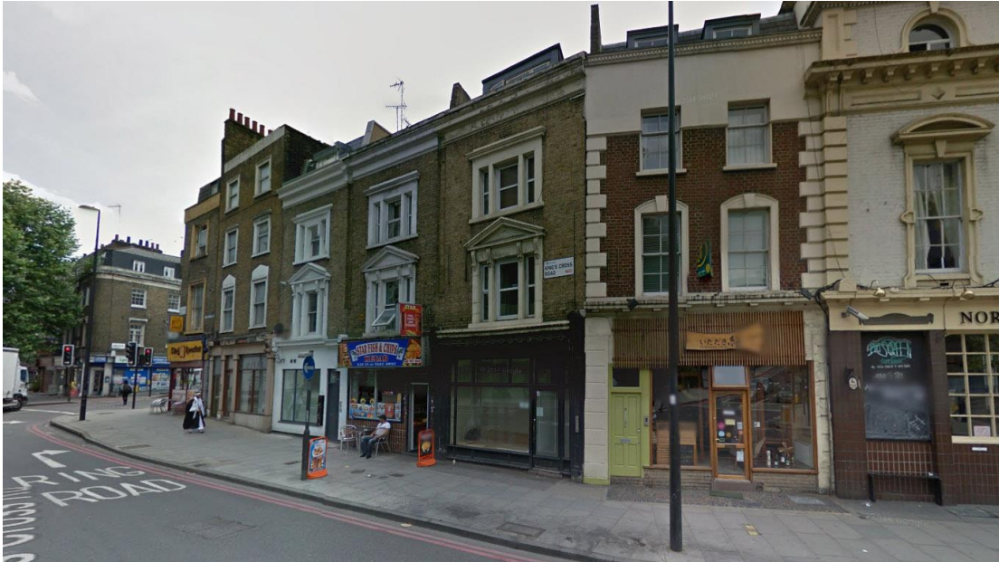
Traditional timber shop front of 137 Kings Cross Road
