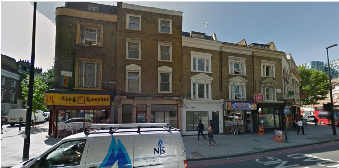
129-137 Kings Cross Road, the row of yellow stock brick houses date to the mid-19th century
