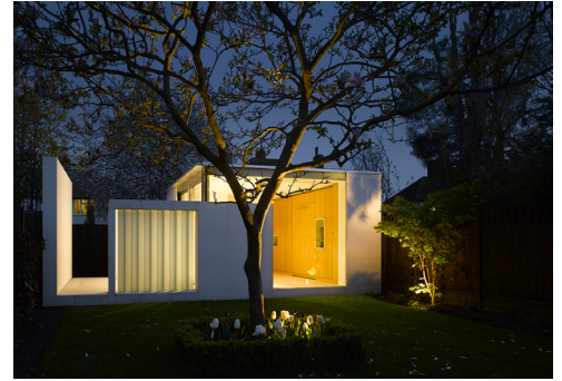
Lonsdale Road Pavilion
