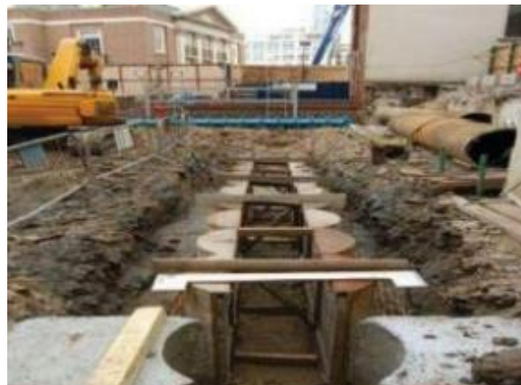
Fig10. Scallops being placed in the trench
