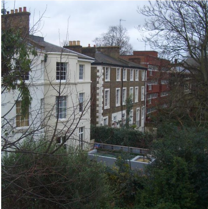
Extension to the rear of Gloucester Avenue
