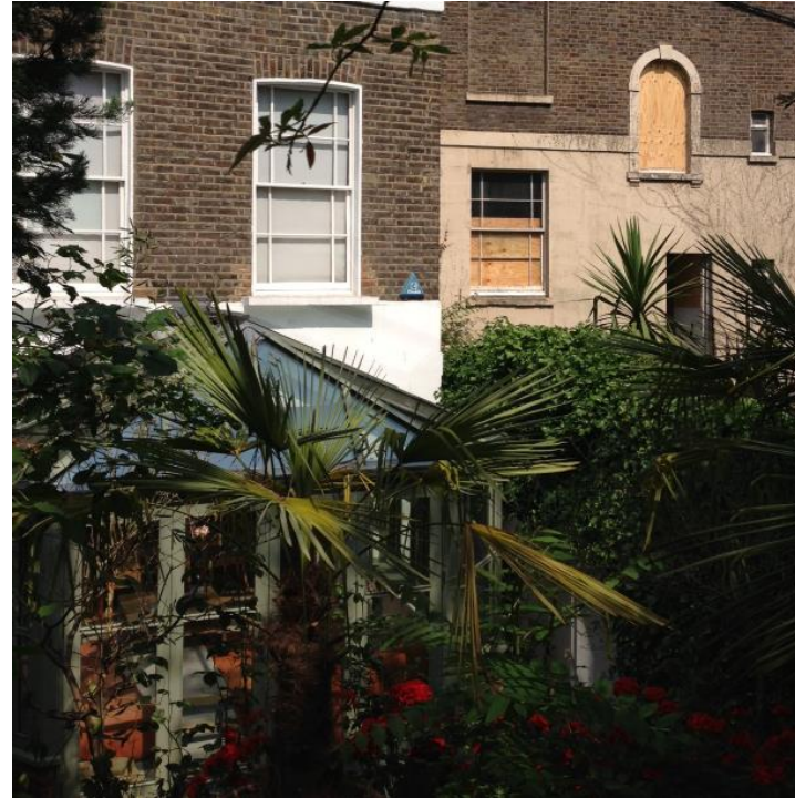
Extension to the rear of 29 St. Mark's Crescent
