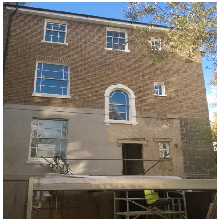
New extension progressing to the rear of No. 30 St. Mark's Crescent
