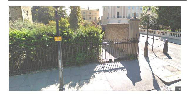
Our proposal is to preserve and reuse all the cast iron that is there in creating the two gates. The older patch plate repairs visible on the gates would be removed and cleaner welds achieved in re-using as much of the old gate as possible. A new vertical post would be made to match the existing gate post and the hinges applied would be made to match the existing gate hinges. All new work would be taken from the original patterns and be of cast iron, painted black, to match the existing.
