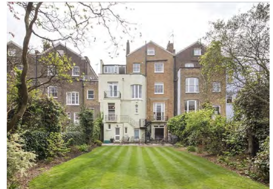
⑥ REAR VIEW 54 REGENT'S PARK ROAD WITH No.52 ON LEFT & No.56 ON RIGHT
