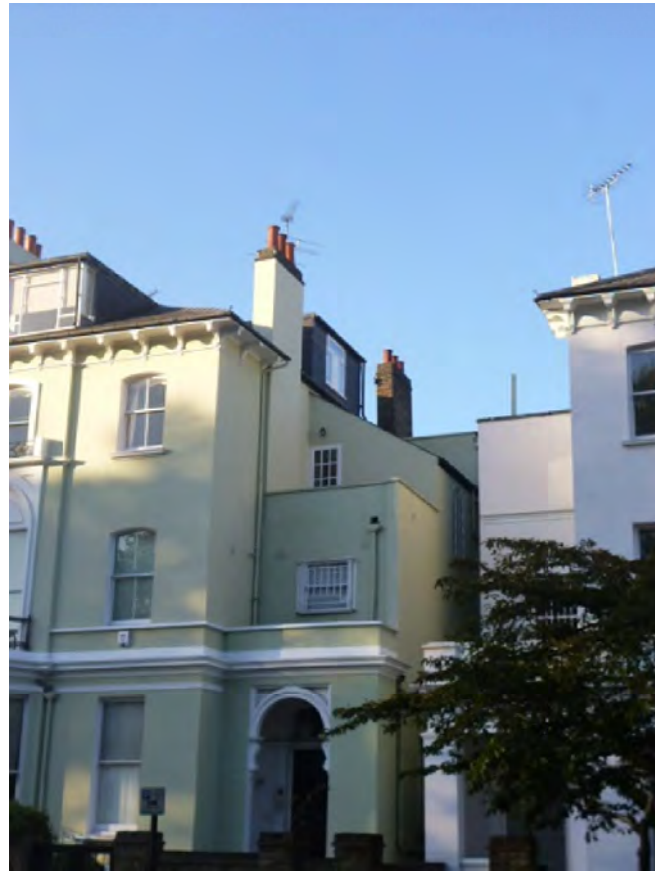
① VIEW OF SIDE WING FROM STREET 54 REGENT'S PARK ROAD
