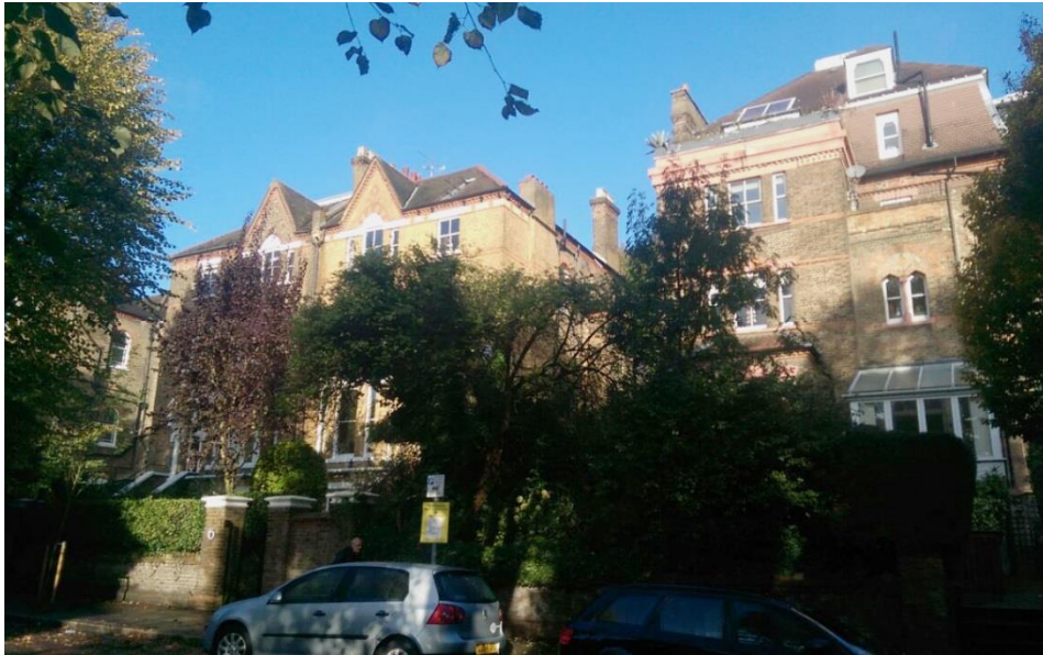
Above: Photograph showing front elevation and surroundings.
