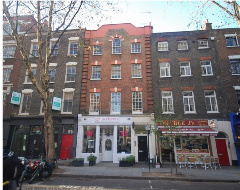
Photograph of 61-65 Charlotte Street as existing
