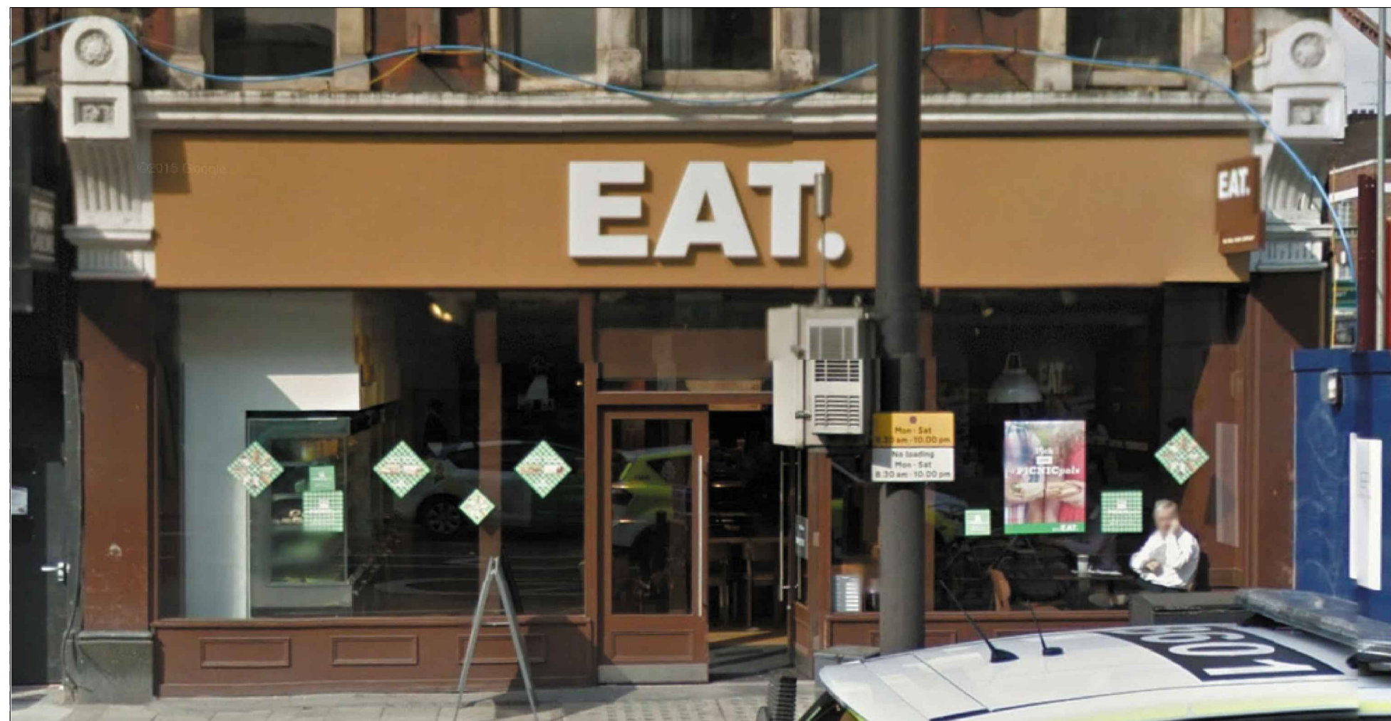
02 62 TCR EXISTING SHOP FRONT STREET SNAPSHOT SCALE: - (A1)
