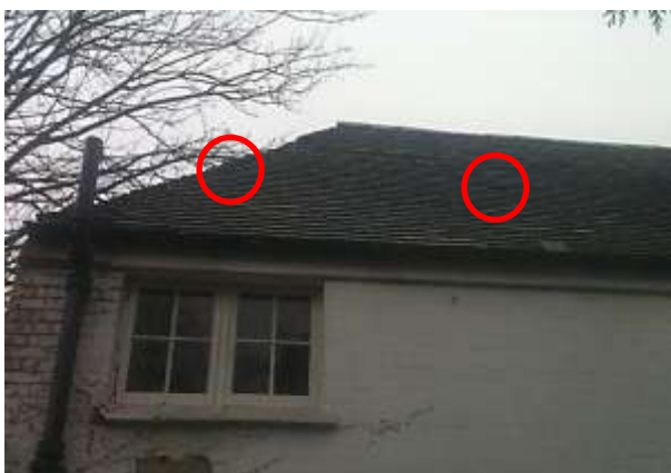
Occasional missing/raised tiles on north west elevation of roof at the rear of the property
