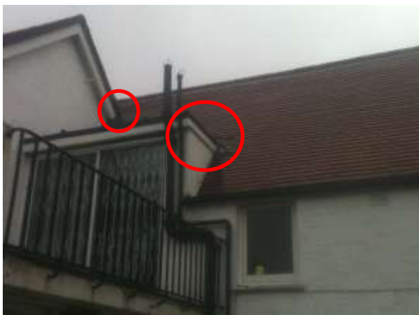
Examples of potential bat access points on the south west elevation of the building, at joins between sections of roofs and also below a fascia board.
