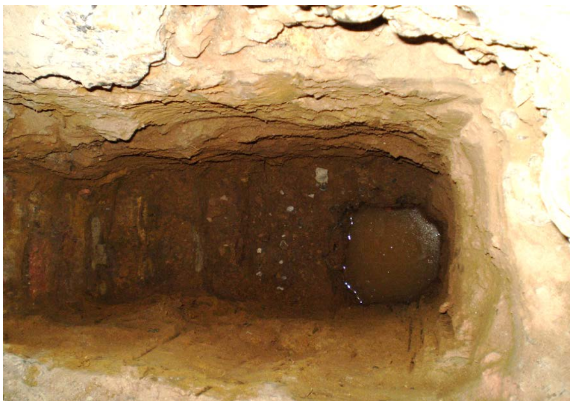
View of the footing encountered in Trial Pit 7 (13/01/2015).
