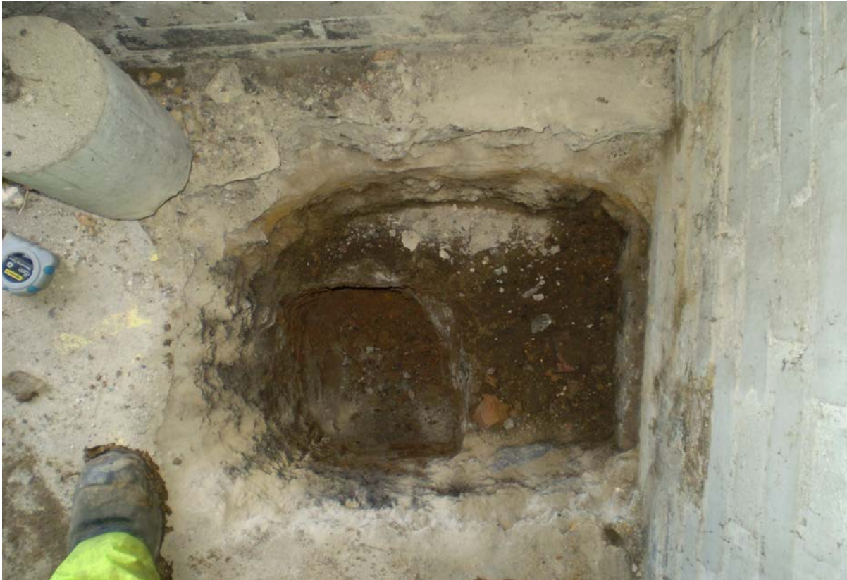
View of the footing encountered in Trial Pit 2 (13/01/2015).
