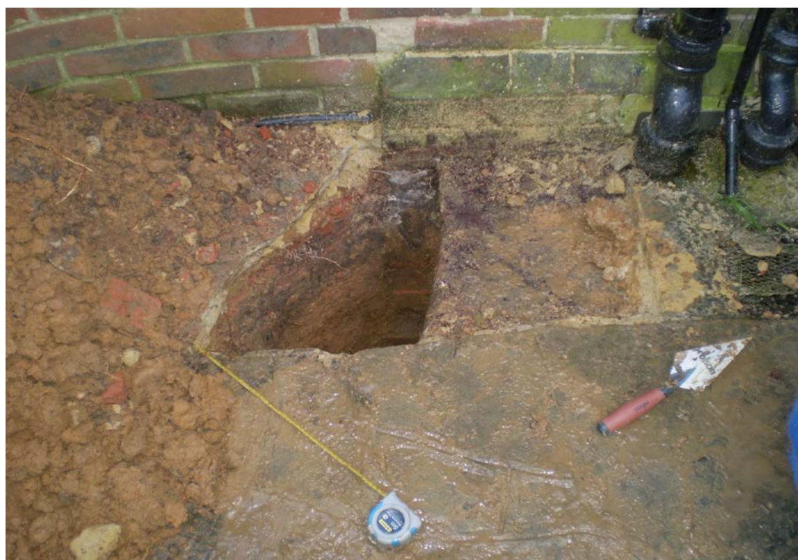
View of the footing encountered in Trial Pit 8 (13/01/2015).
