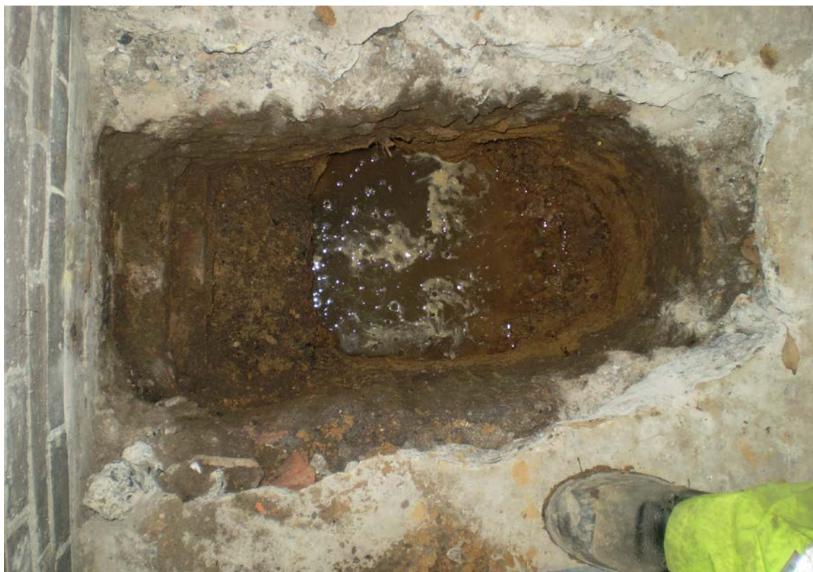
View of the footing encountered in Trial Pit 9 (13/01/2015).
