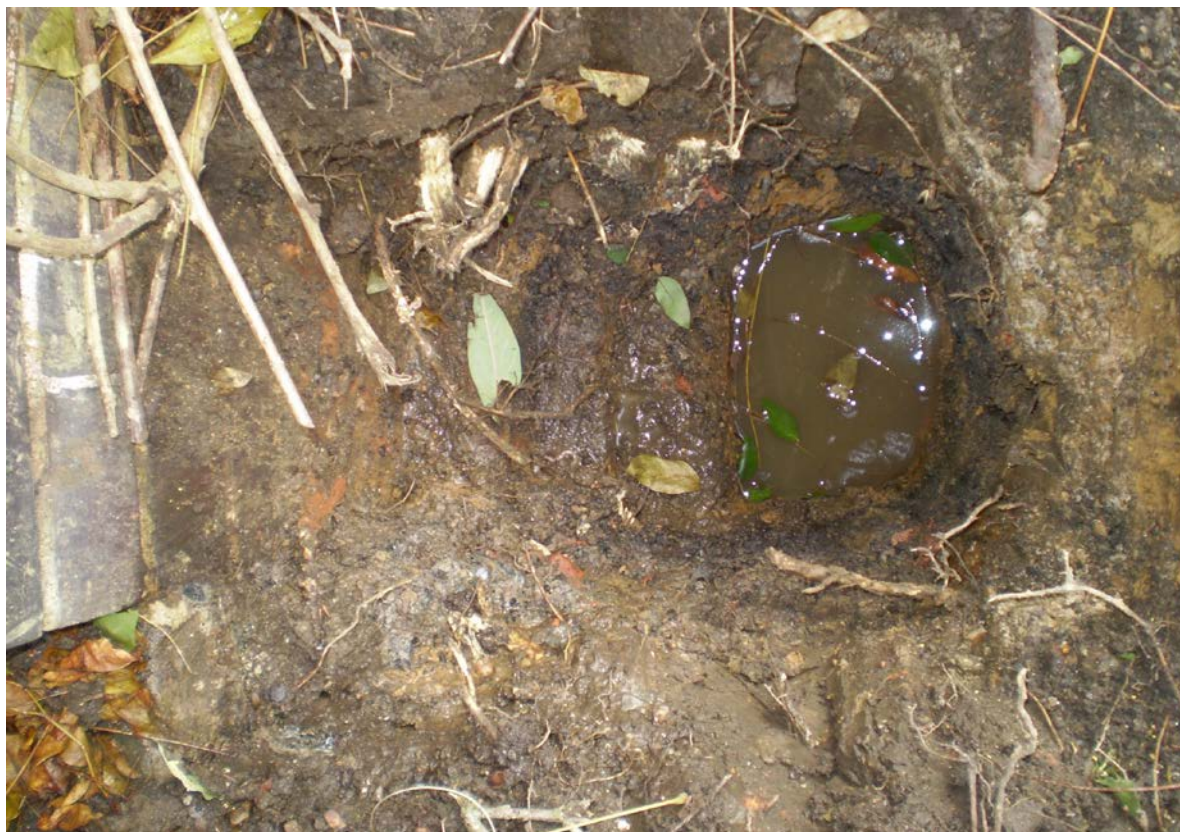
View of the footing encountered in Trial Pit 6 (13/01/2015).
