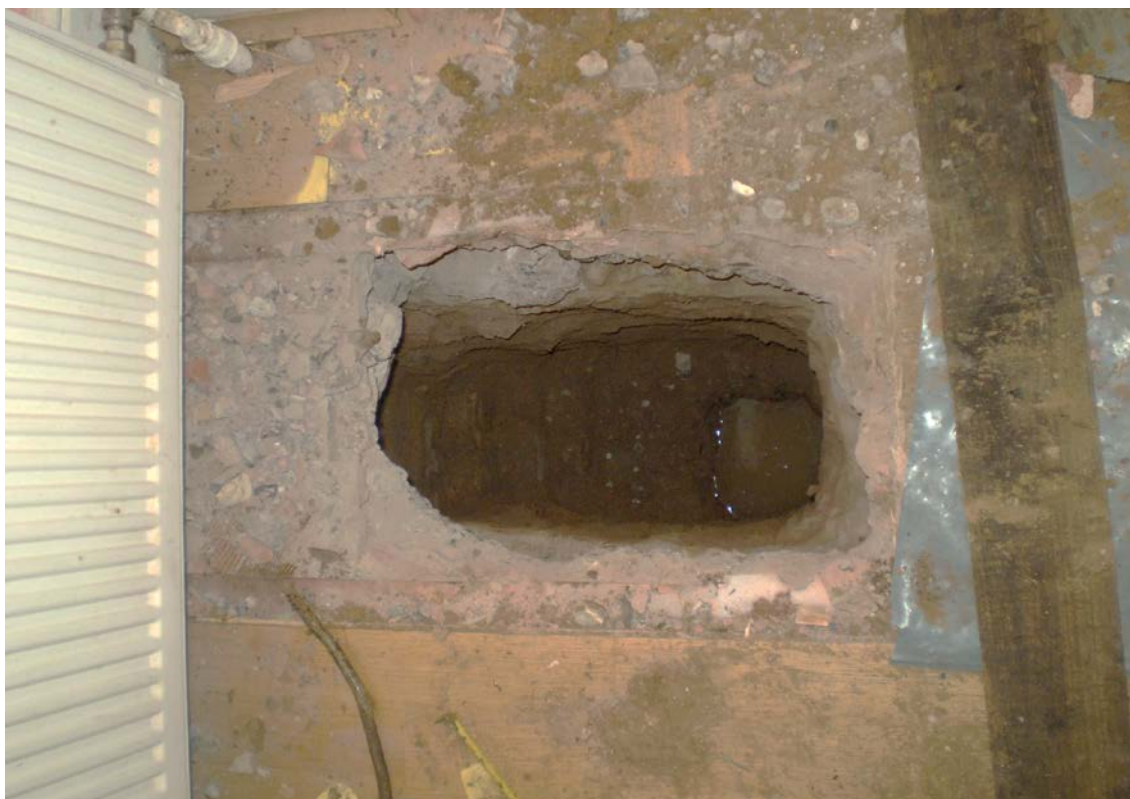
View of the footing encountered in Trial Pit 7 (13/01/2015).
