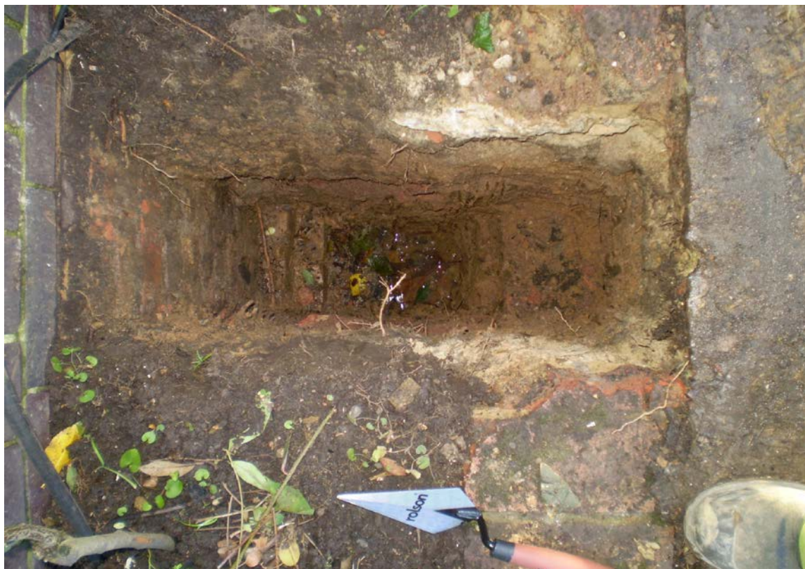
View of the footing encountered in Trial Pit 3 (13/01/2015).
