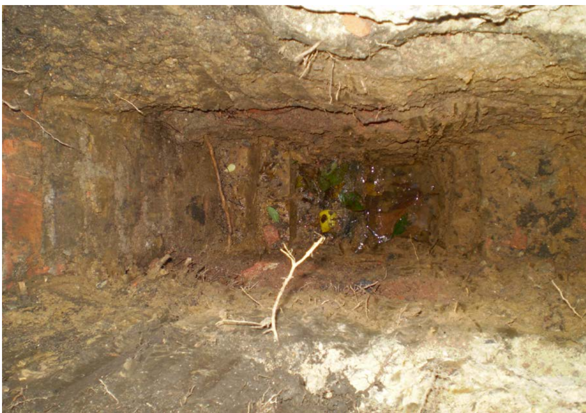
View of the footing encountered in Trial Pit 3 (13/01/2015).
