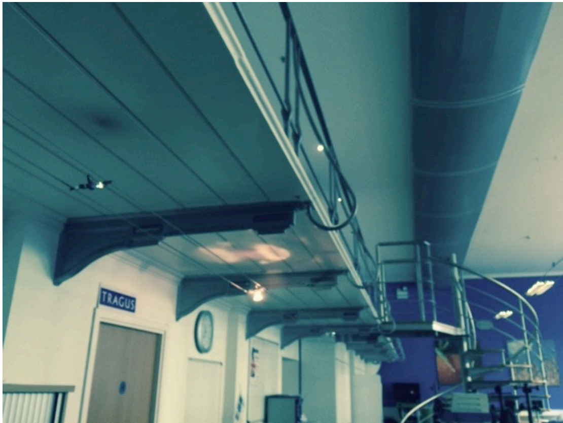
Fig. 11 Current photograph of rear gallery and recently installed spiral stair
