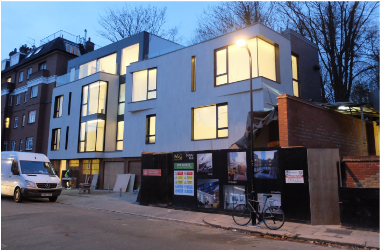
Photo 2: Development near completion
