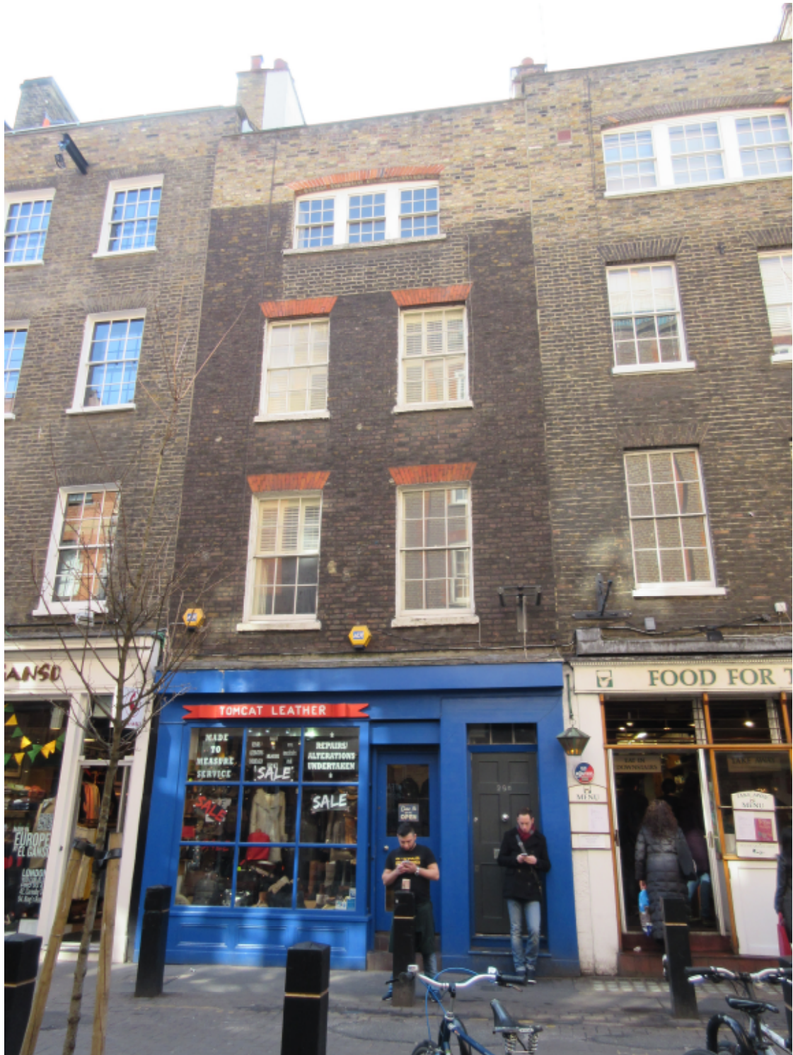
Front elevation of subject property, also showing relationship with 27 and 31 Neal Street
