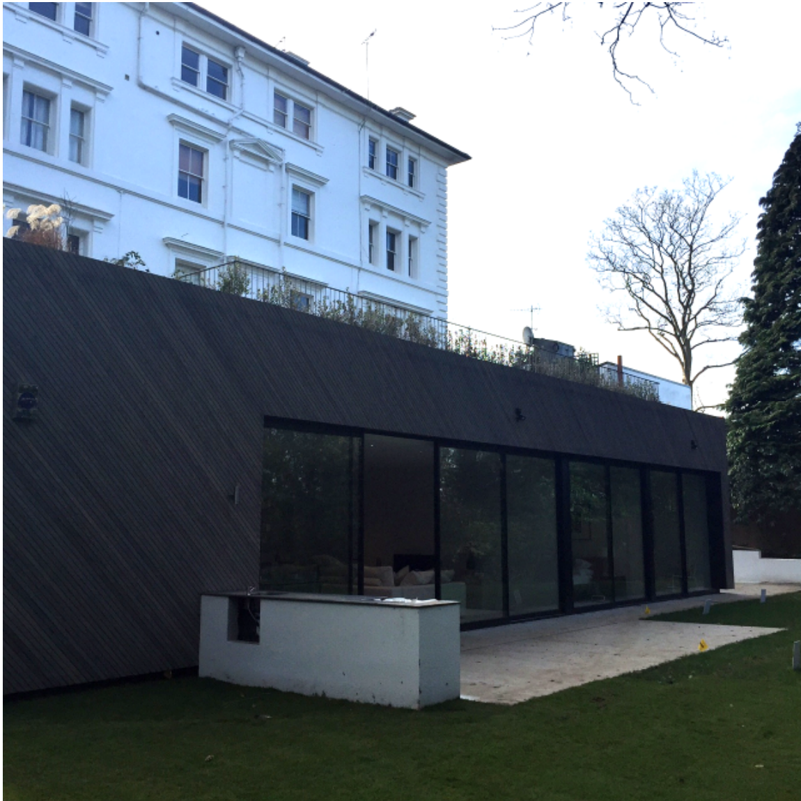
Photo 1 – New dwelling as built, garden facing elevation
